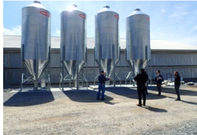
⬆ Feed bins installation at the ETREC-Little River Unit freestall barn
