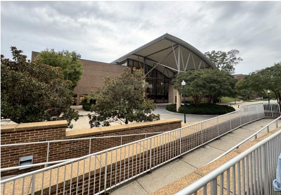
20 View looking at the University Center and existing ADA ramp to be demolished
