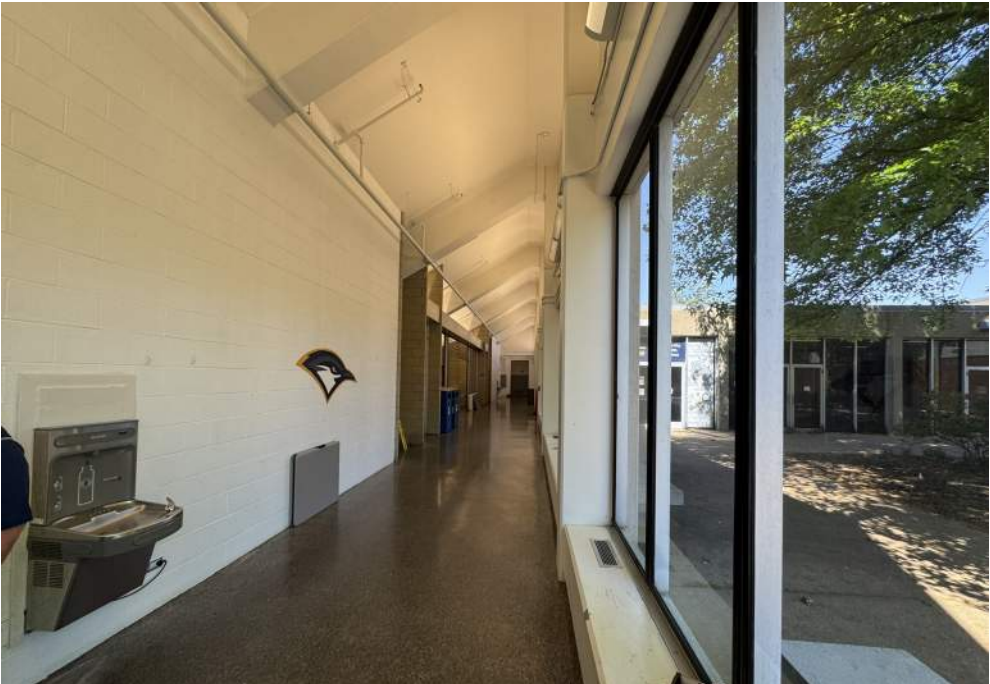
14 View looking at the existing concourse corridor
