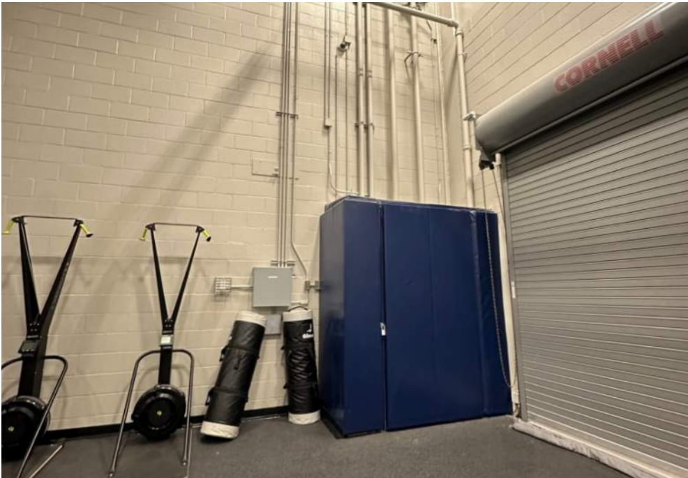
10 Existing electric panel and roll-up door at wrestling space
