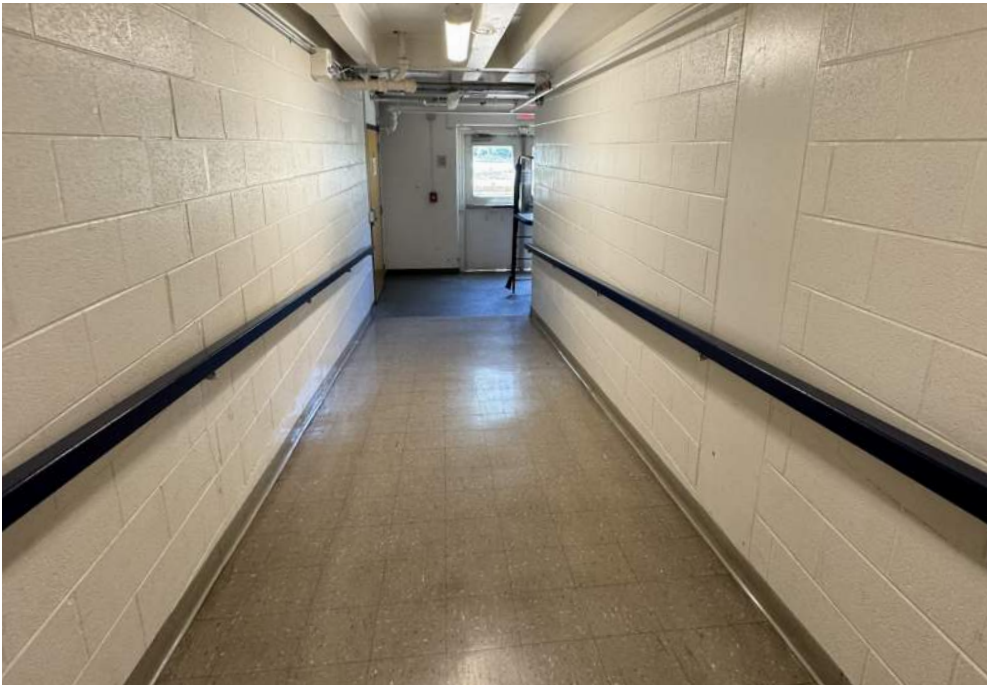
11 Existing ramp connecting the south entry and gym level
