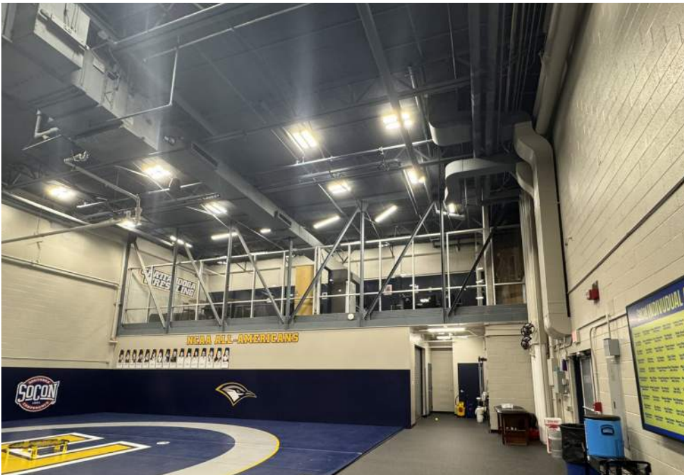
8 View looking at wrestling space
