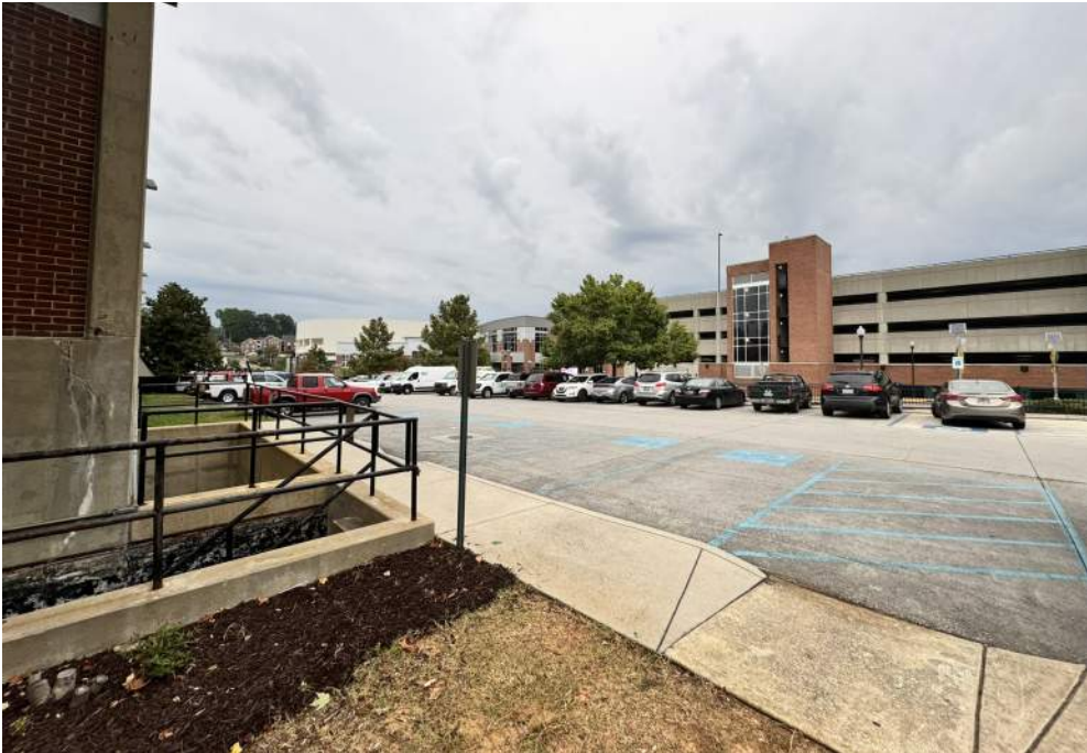
17 View looking at the existing parking lot, to be demolished
