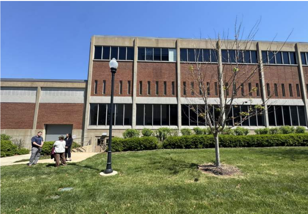
21 View looking at the south facade, existing gym
