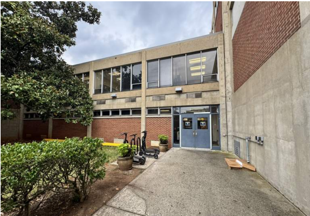
1 View from Douglas Street
