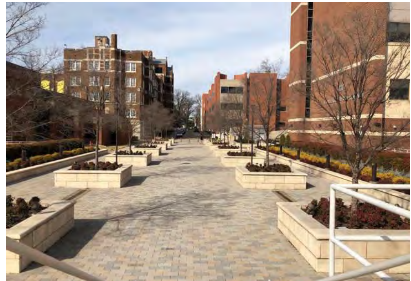
Pedestrian Extension at Monroe Avenue
